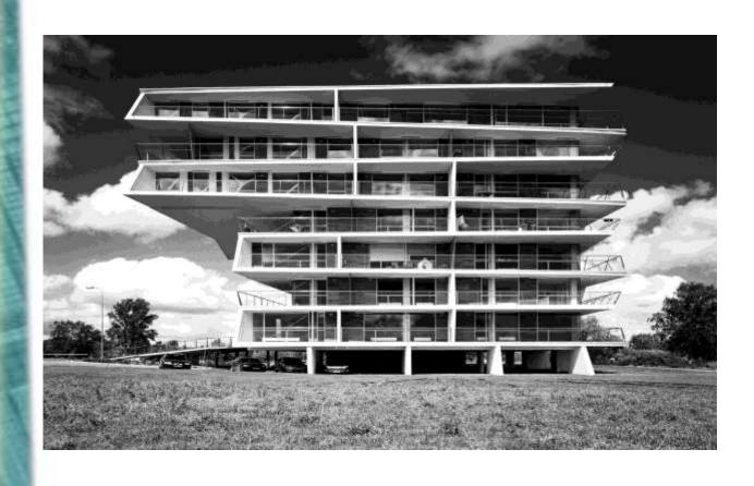
Free facade was a consequence of concrete frame construction. Because walls were then deprived of their constructional role, their design became free as well.
